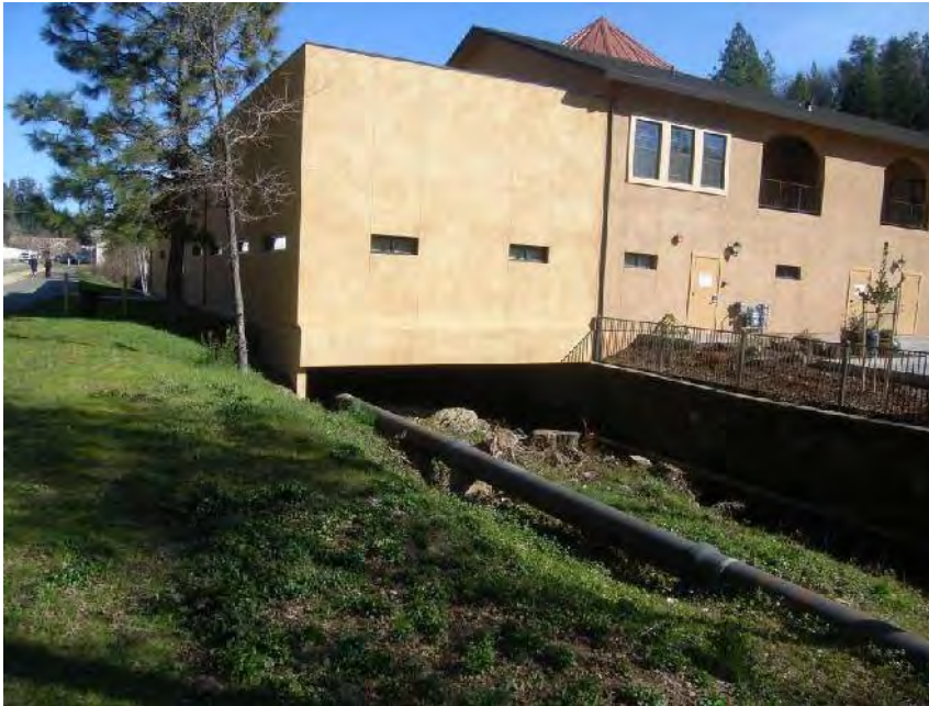
Photograph 1: Building near Locust Avenue
